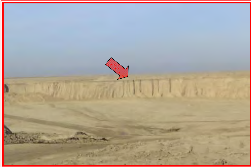
Photo No. 13 : Vertical Cuts at borrow pit at km 269+500
