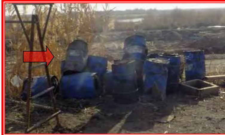
Photo No. 8 : Improper hazardous waste management (spills and drums) at bridge no. 1 Subcontractor camp
