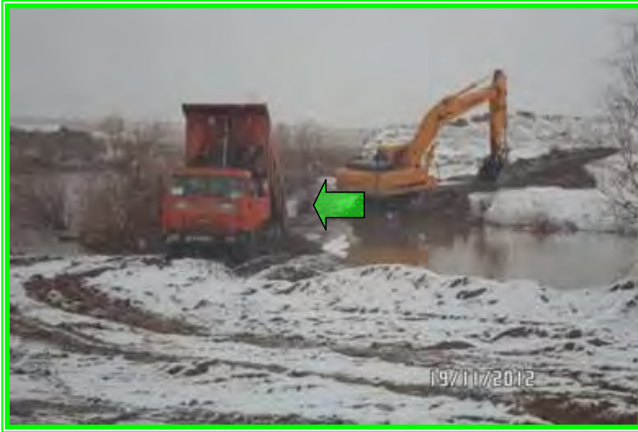
Photo No. 3 : Contractor starting to increase the elevation of filter berm
