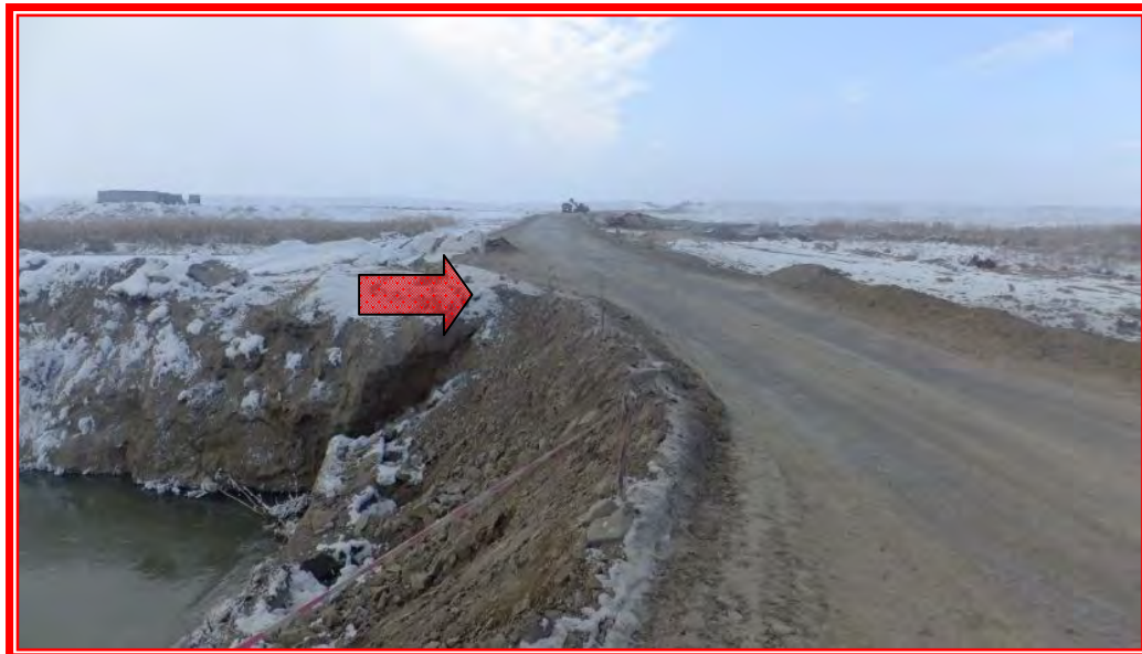
Photo No. 12 : Unchanged situation at bridge no. 3
