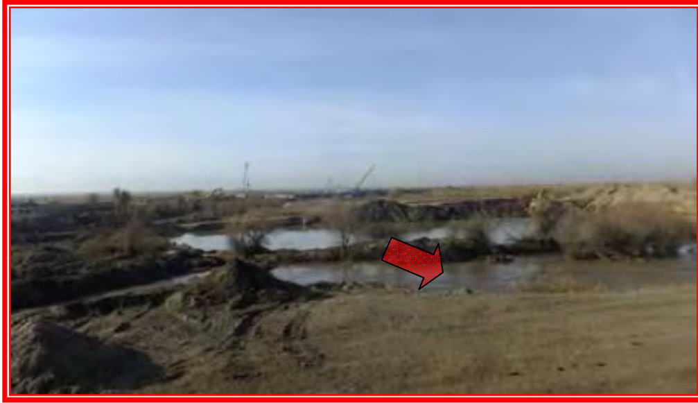
Photo No. 1 : Pond's silt holding capacity near spilling condition
